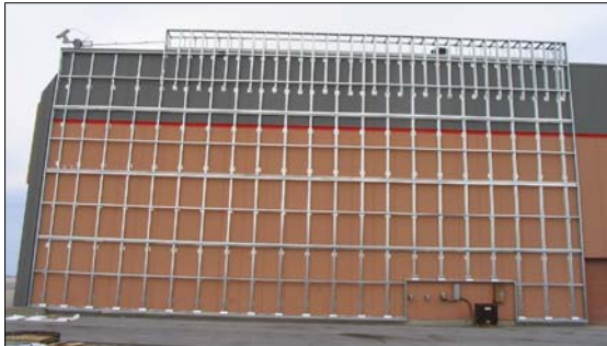
Above, the SolarWall framing
