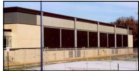
Breck School, Minneapolis, Minnesota
